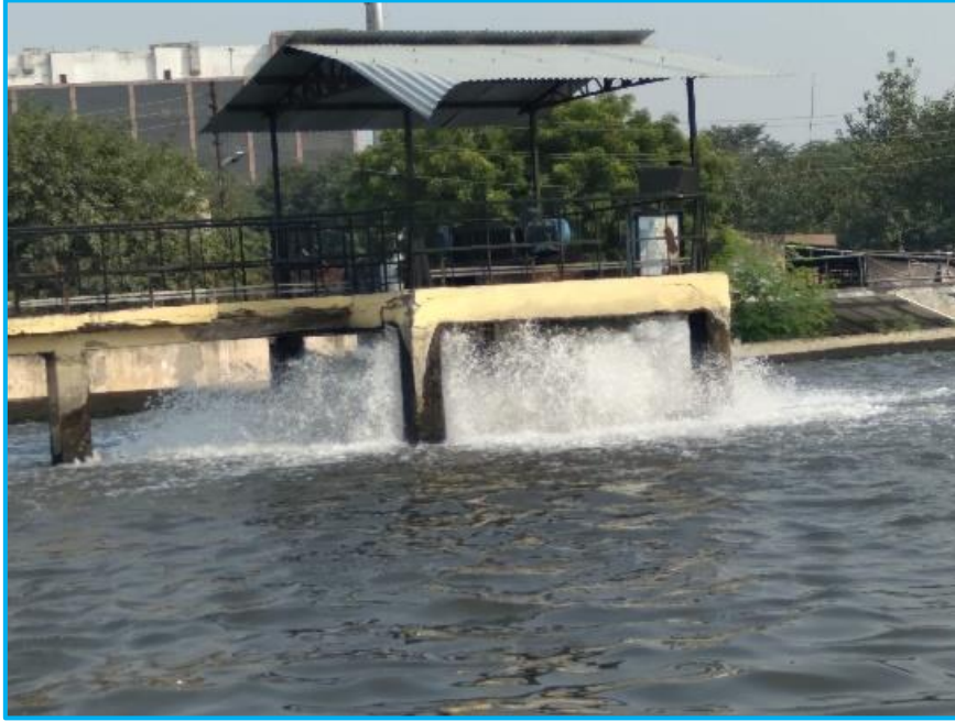
Sewage Treatment Plant
